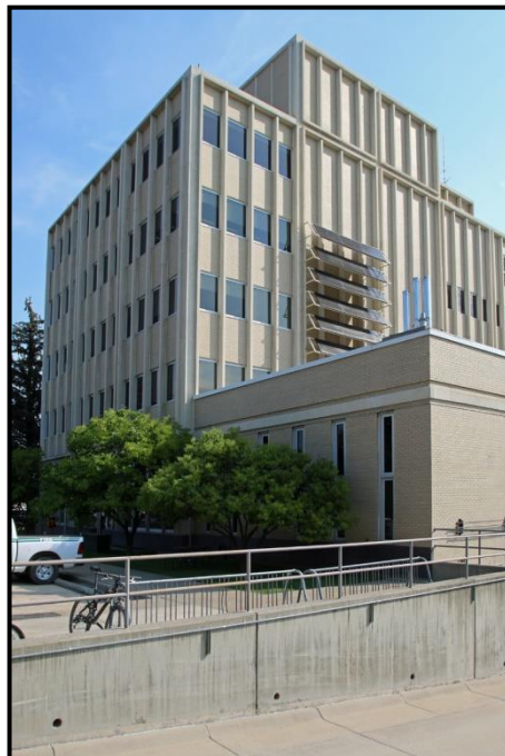
Photograph 4. Overview of the west elevation, facing northeast.
