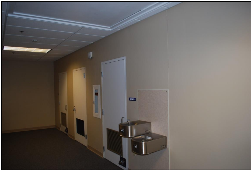
Photograph 20. Widened fifth-floor restroom entries, facing southwest.
