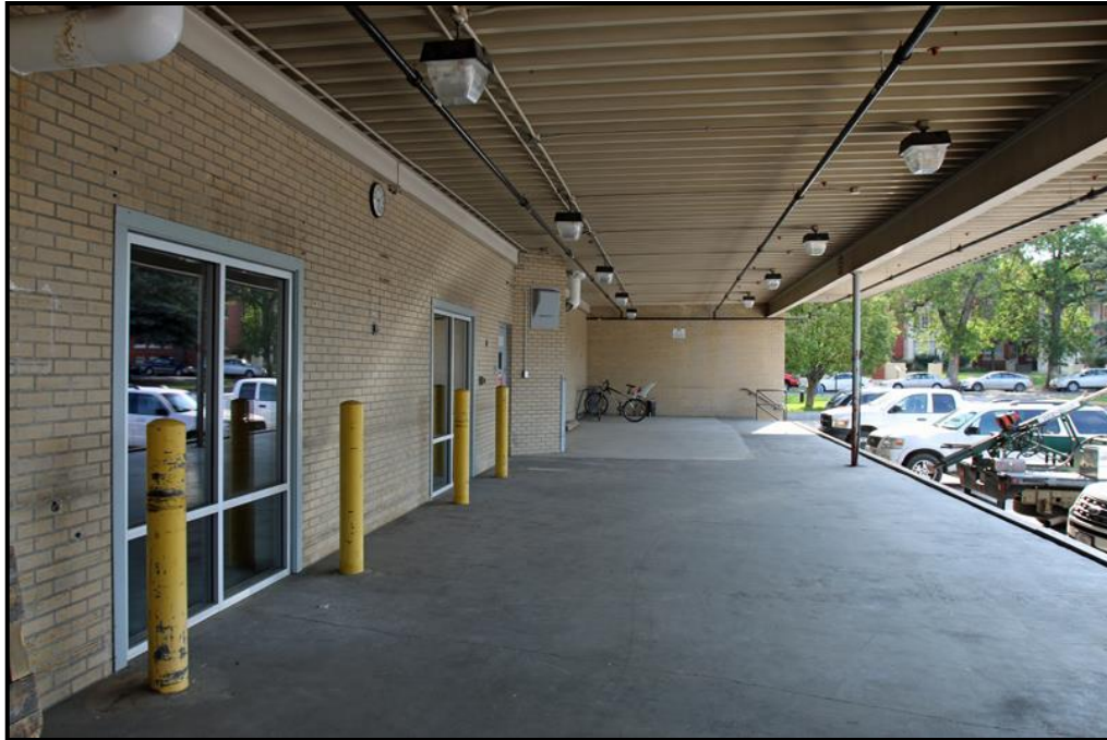
Photograph 7. Overview of the loading platform, facing east.
