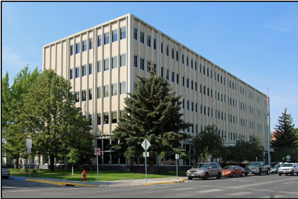
Photograph 1. Overview of the FB&USPO, facing southwest.
